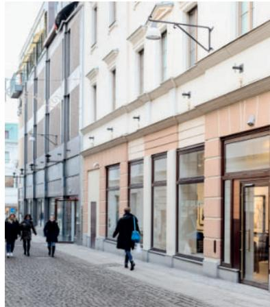
ty. The first project to be carried out involved moving the line of the building out to the facade plane, with the result that the existing arcades on the ground floor have been enclosed. This generated more floor space in the department store and created an entrance directly from the street for the new stores. By doing so, a more pleasant and safer urban space was established, which also helped to reinforce the whole of the Fredstan retail area. The project was completed during the year.
