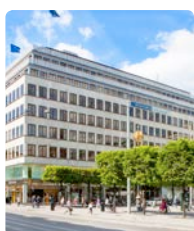
Packarhuset 4 Construction year: 1932 Rentable space: 15,399 sq m
