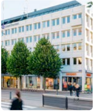
Nordstaden 8:24 (Fyran) Construction year: 1972 Rentable space: 21,201 sq m
