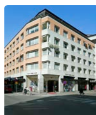
Skären 9 Construction year: 1984 Rentable space: 11,003 sq m
