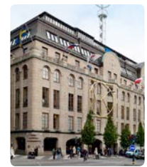
Hästen 19 (NK) Construction year: 1915 Rentable space: 39,406 sq m
